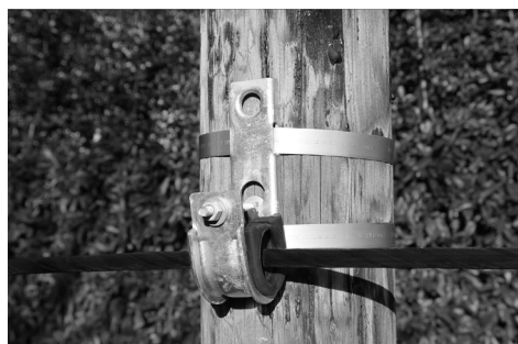
Fixing with 2 steel straps 20 x 0,7 or 0,4 mm
